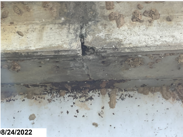
Delam & Spalling in Overhang Span 1 Rt. Side at Saw Joint.
