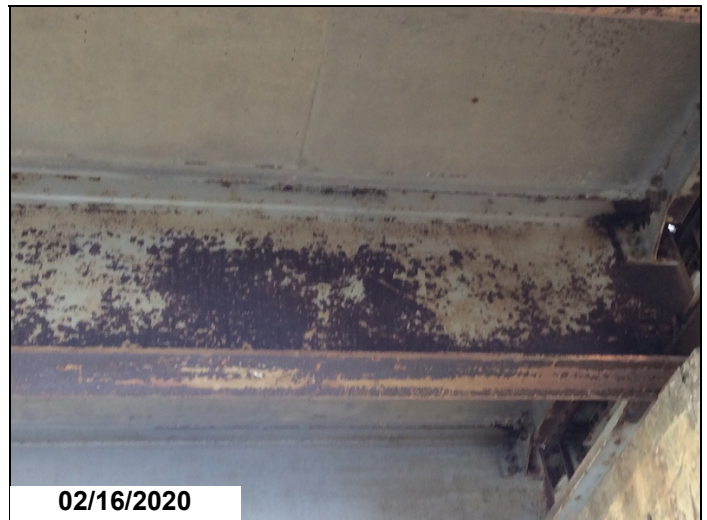
Typ. Rust on Beams.
