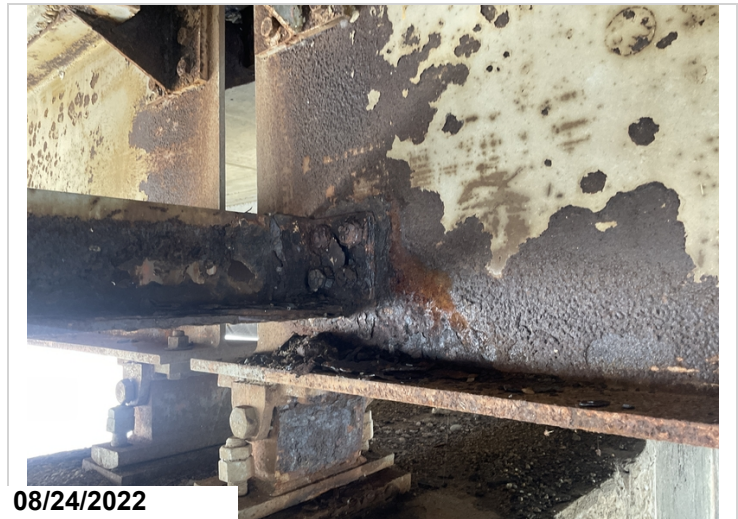
Typ. Rust & Section Loss on End of Beam 3 Pier 5 Bk. Side. Up to 3/8" Section Loss on Lower Web at Diaphragm Connection
