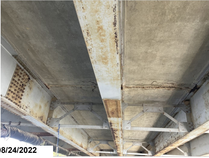
Typ. Condition of Soffit.
