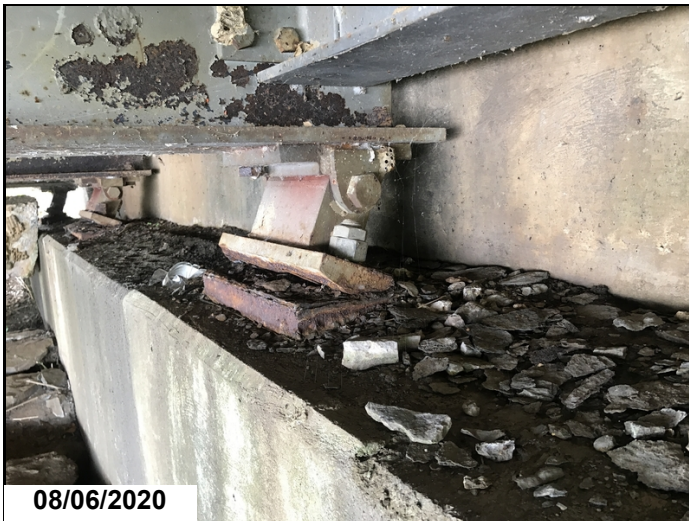
Bent 1 bearings are full of pack rust and are fully tilted.
