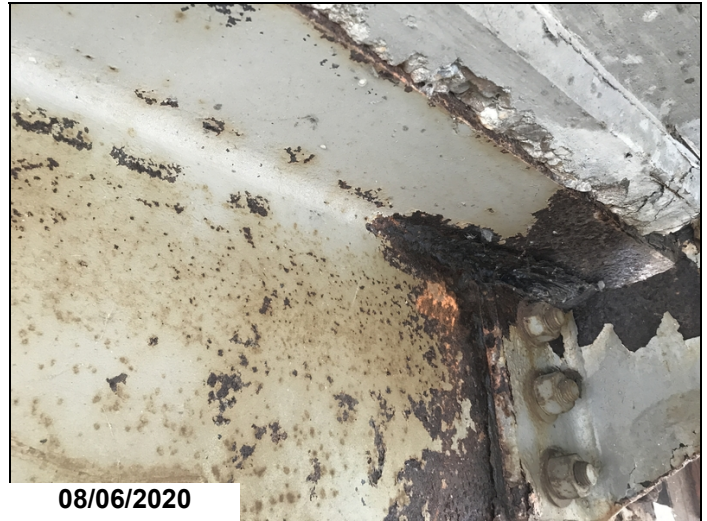
Bent 5 span 4 girder 3 has approximately 1/4" section loss in the haunch area. The web is 5/8" thick. Also web at diaphragm connection has 3/16" section loss.
