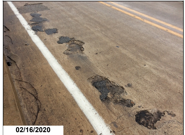
Typ Patched Areas & Spalling in Deck.
