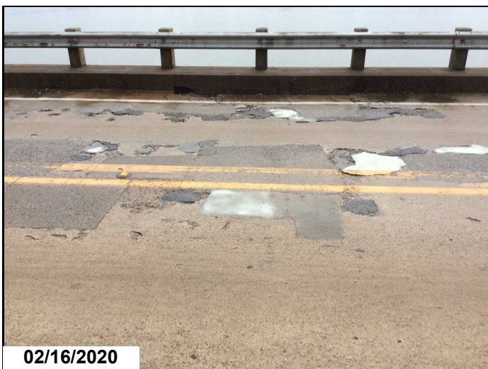
Typ. Patched Areas & Spalling Areas in Deck.
