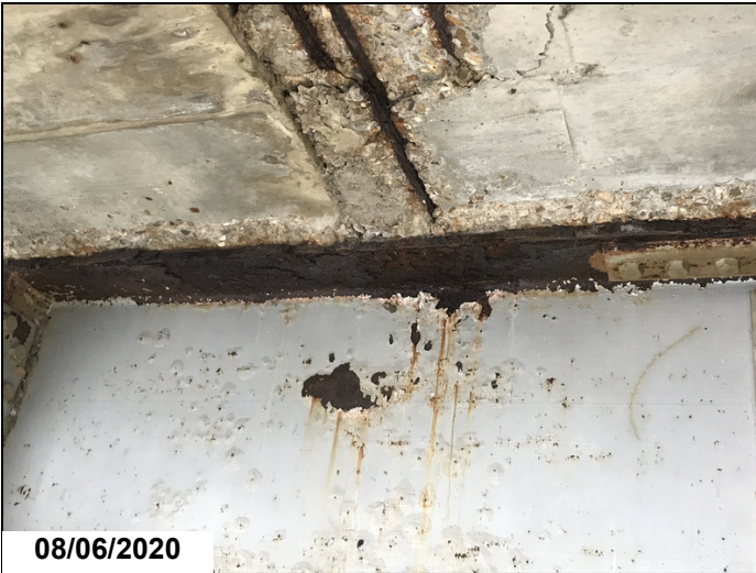
Span 4 girder 5 has moderate section loss in top flange at the first splice plate.
