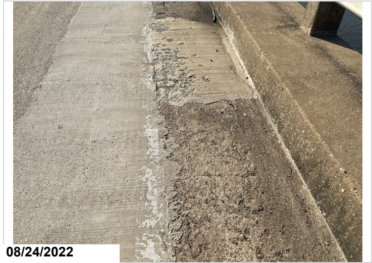
Typ. Scale in Gutters & Patched Areas in Gutters. Rt. Side. Spans 3 & 5.
