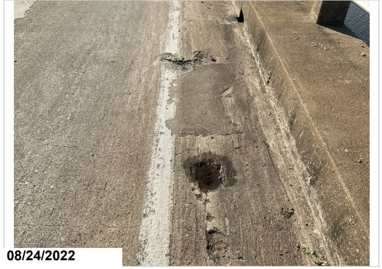
Typ. Delam & Spalling in Gutter. Rt. Side.
