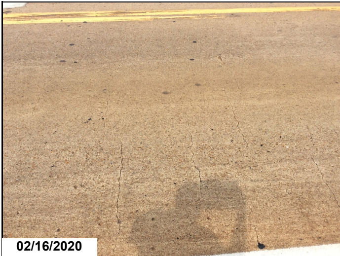
Typ. Cracking in Deck.
