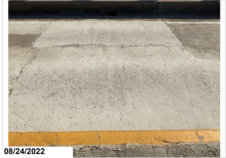
Typ. Cracking in Patched Areas. Span 8
