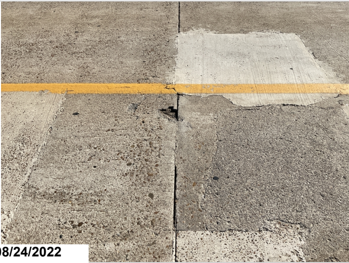
Typ. Delam & Spalling at Saw Joints in Span 7.
