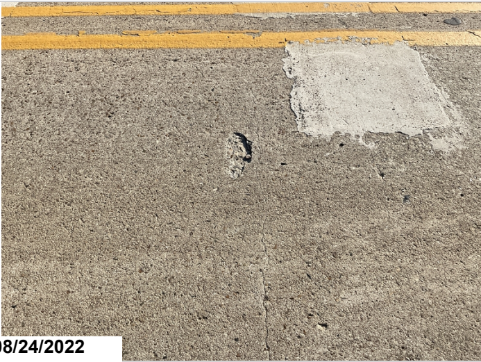
Typ. Delam & Spalling in Deck.
