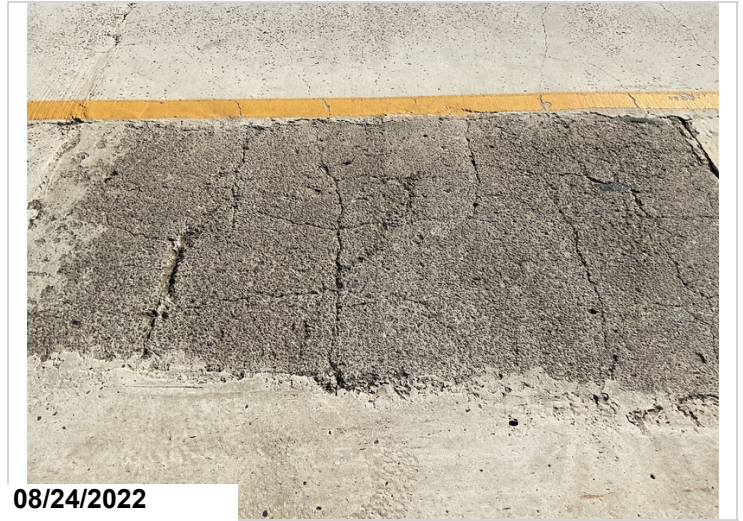
Typ. Condition of Old Patches. Span 8
