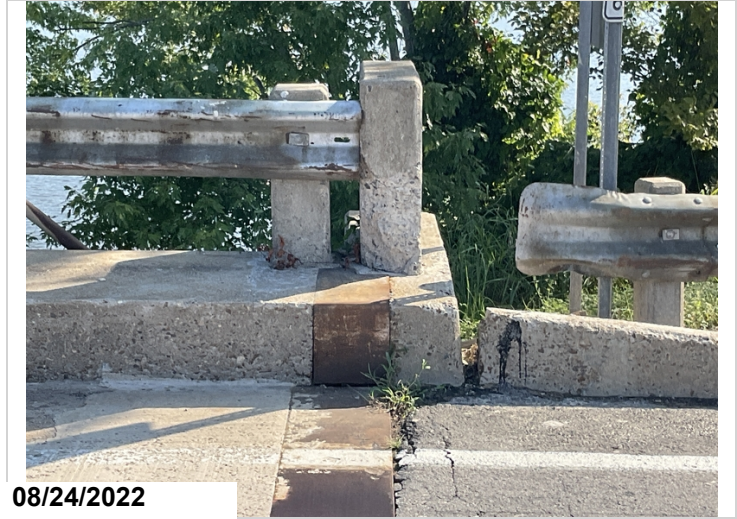
Impact Damage to Rail & Post at Abutment 9 Lt. Side.
