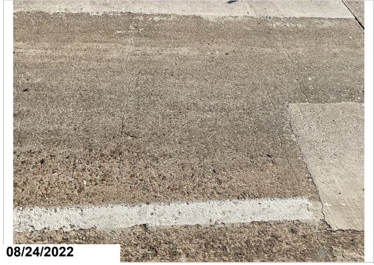
Typ. Cracking in Deck.
