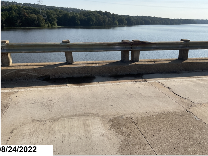
Impact Damage to Rail & Post at Pier 7 Lt. Side.
