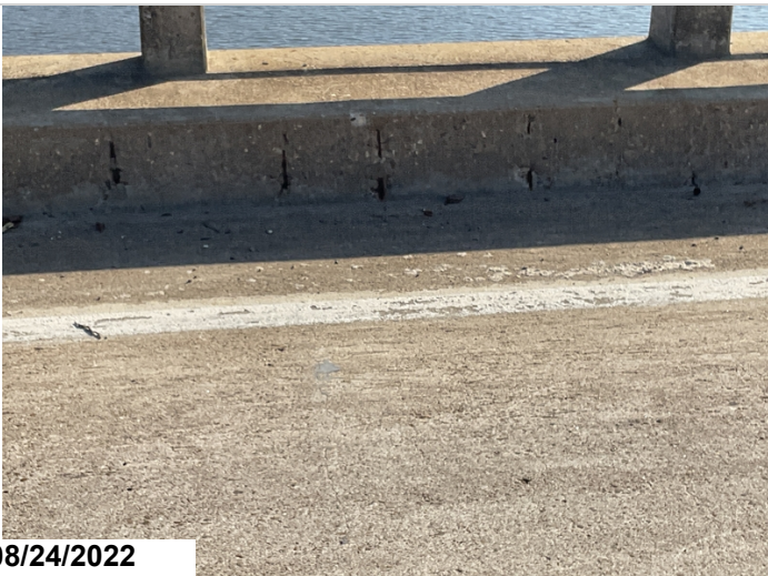
Typ. Delam & Spalling W / Rebar Exposed in Curbs.
