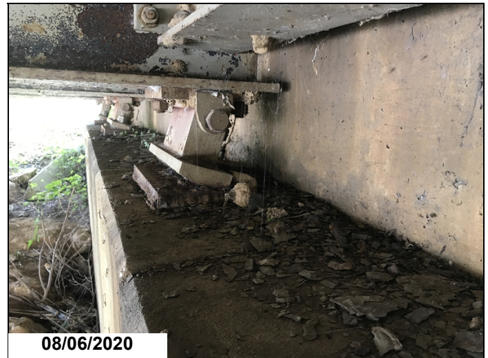
Moveable bearings at bent 8 are fully extended.
