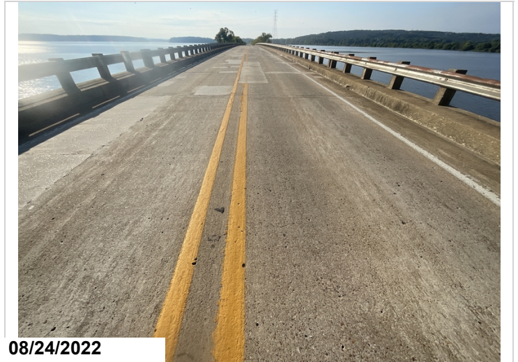
Typ. Condition of Deck.
