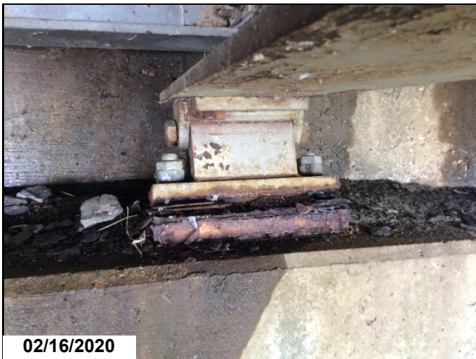
Typ. Rust on Bearings.
