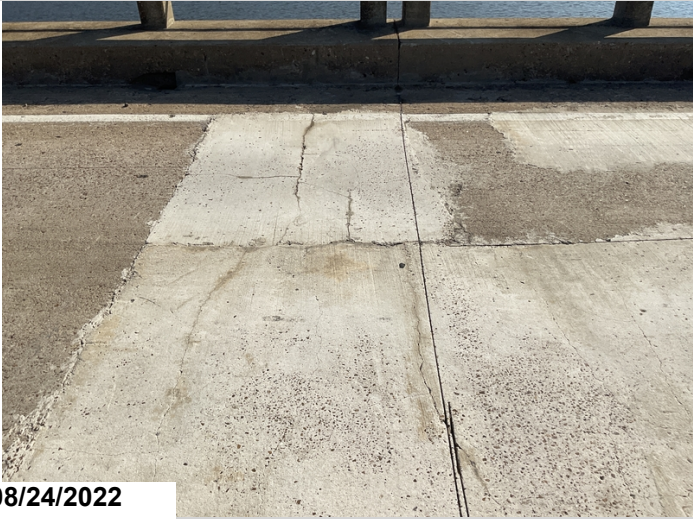
Typ. Cracking in Patched Areas. Span 8
